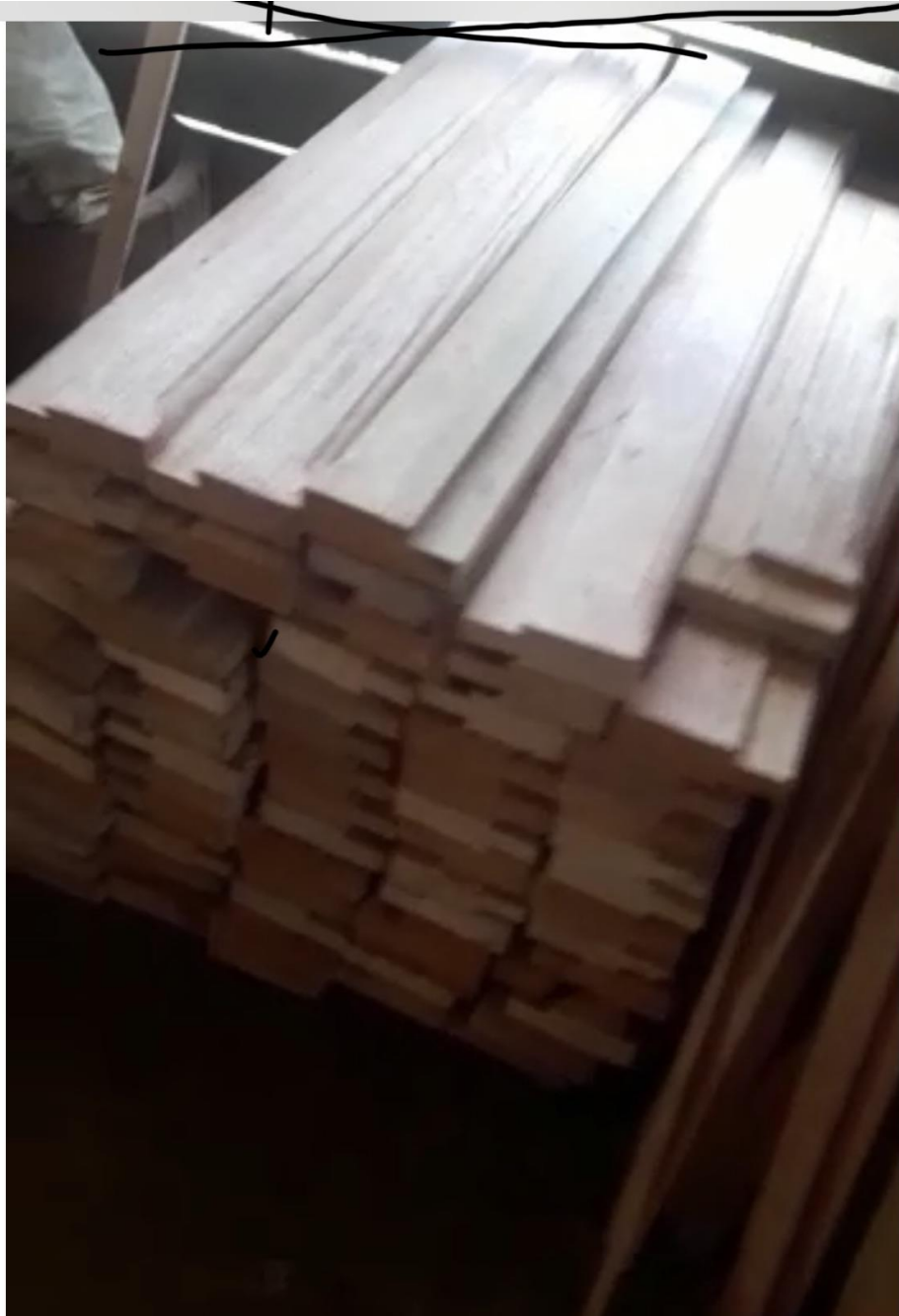
Frames for 16 window and 2 doors, to be assembled at the site of project
