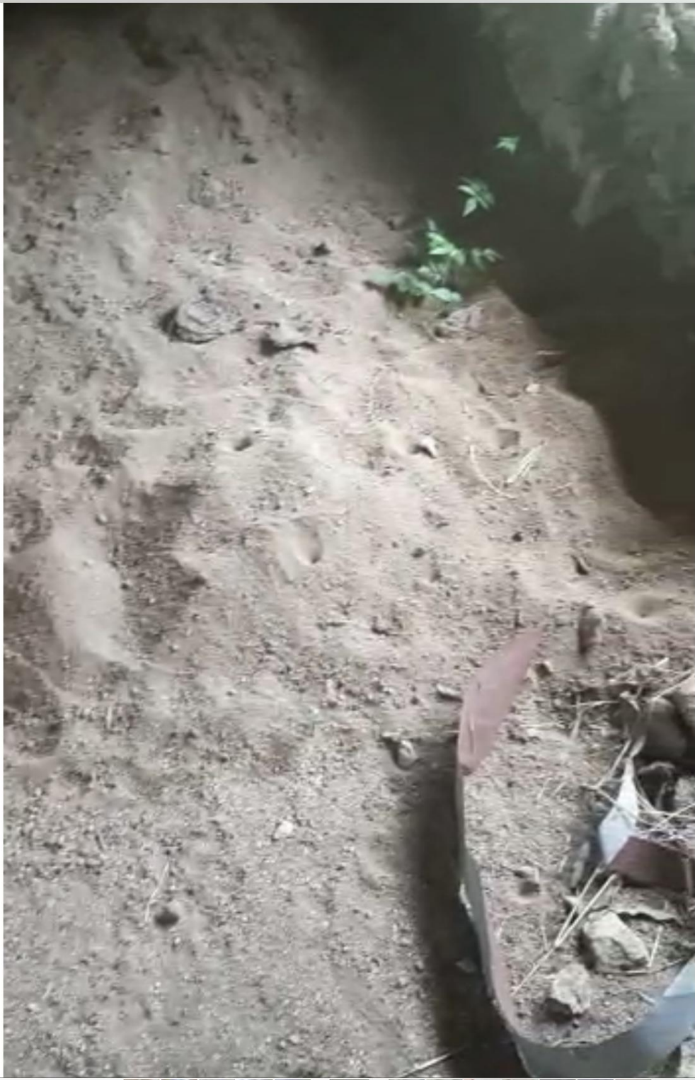
Sand at the construction site
