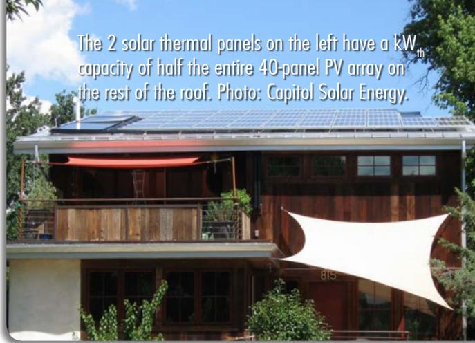
The 2 solar thermal panels on the left have a kW<sup>th</sup> capacity of half the entire 40-panel PV array on the rest of the roof. Photo: Capitol Solar Energy.
