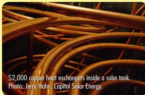
\$2,000 copper heat exchangers inside a solar tank.
