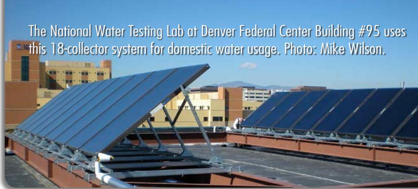
The National Water Testing Lab at Denver Federal Center Building #95 uses this 18-collector system for domestic water usage. Photo: Mike Wilson.
